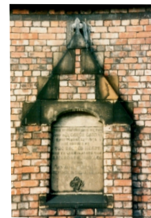
Old Junior School Foundation Stone
