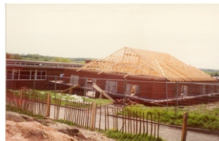
Junior Extension Building under construction 1996
